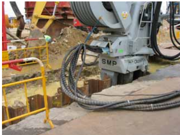
Specially designed equipment for noise protection
