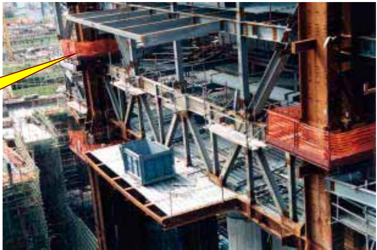
Detail of the south elevation of the transfer truss
