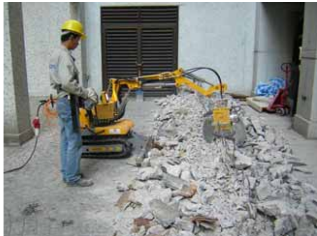
Specially designed crusher for better noise protection
